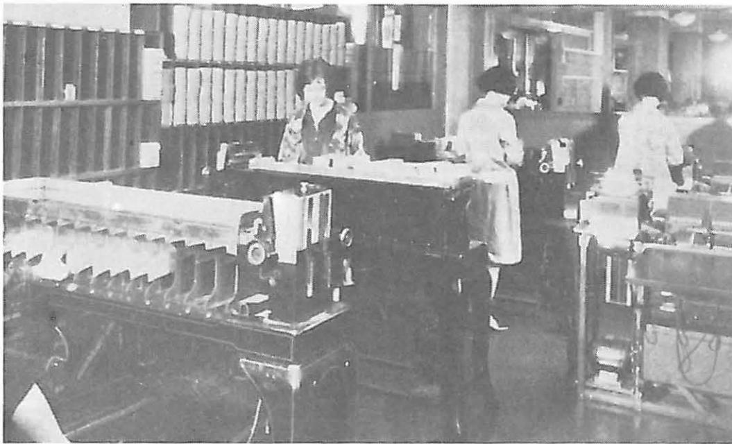
*Hollerith punch-card equipment as used in 1931 to mechanize and simplify paperwork.*
