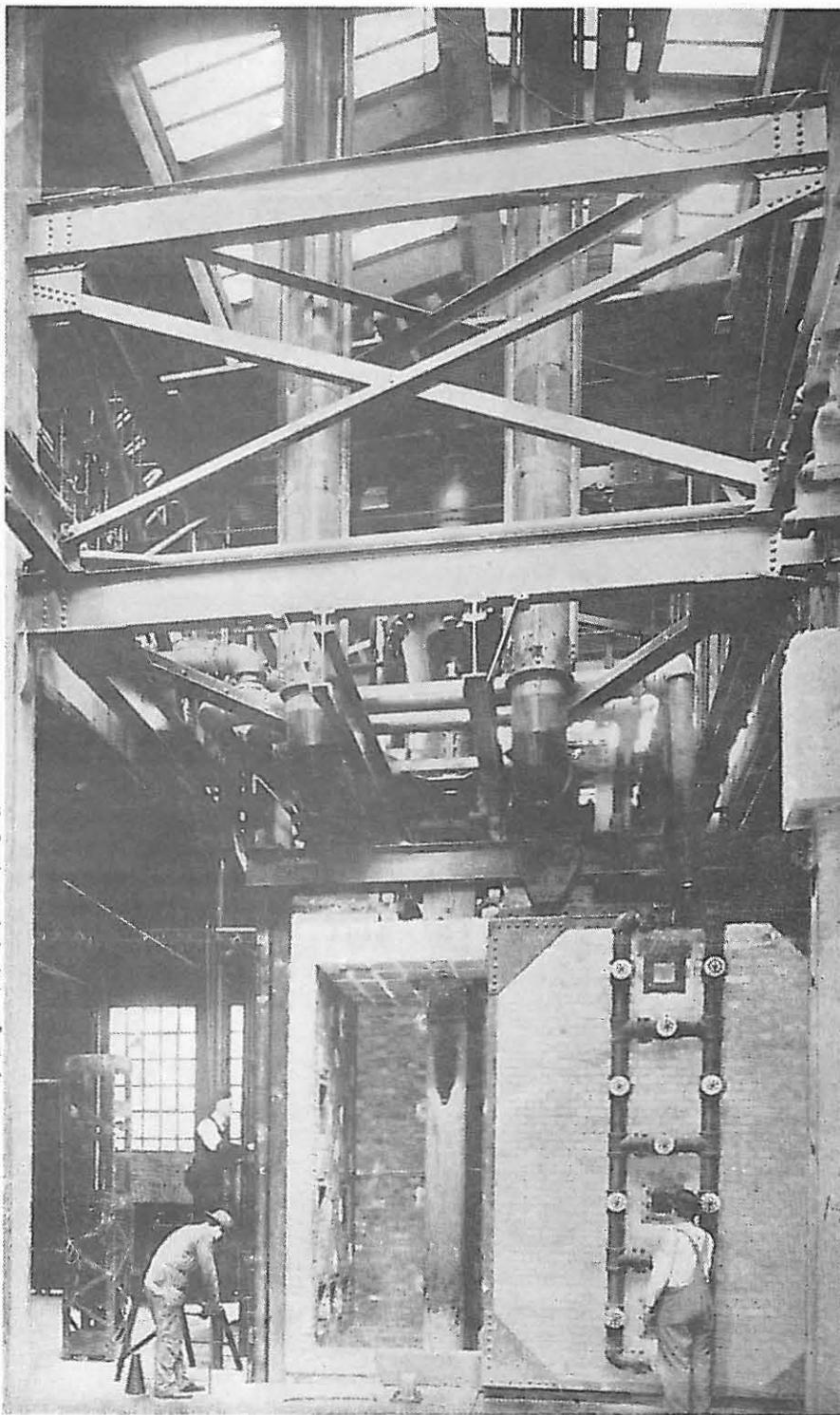
*The CFUA utilized data from the Underwriters Laboratories. Here in the Chicago facility a ponderous structure was built to test fireproof columns.*
